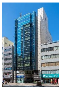
Hiroshima Rijo-dori Building (Implemented within the reporting period)
