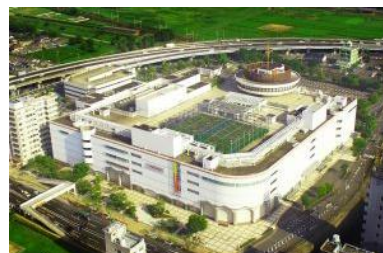
Mi-Nara (building perimeter exterior lights) (Implemented within the reporting period)
