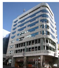
MI Terrace Kita-Ueno (Some private areas and emergency lighting) (Implemented within the reporting period)
