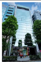
MI Terrace Yokohama Nishiguchi
