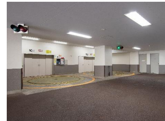
Parking garage (64 cars)
